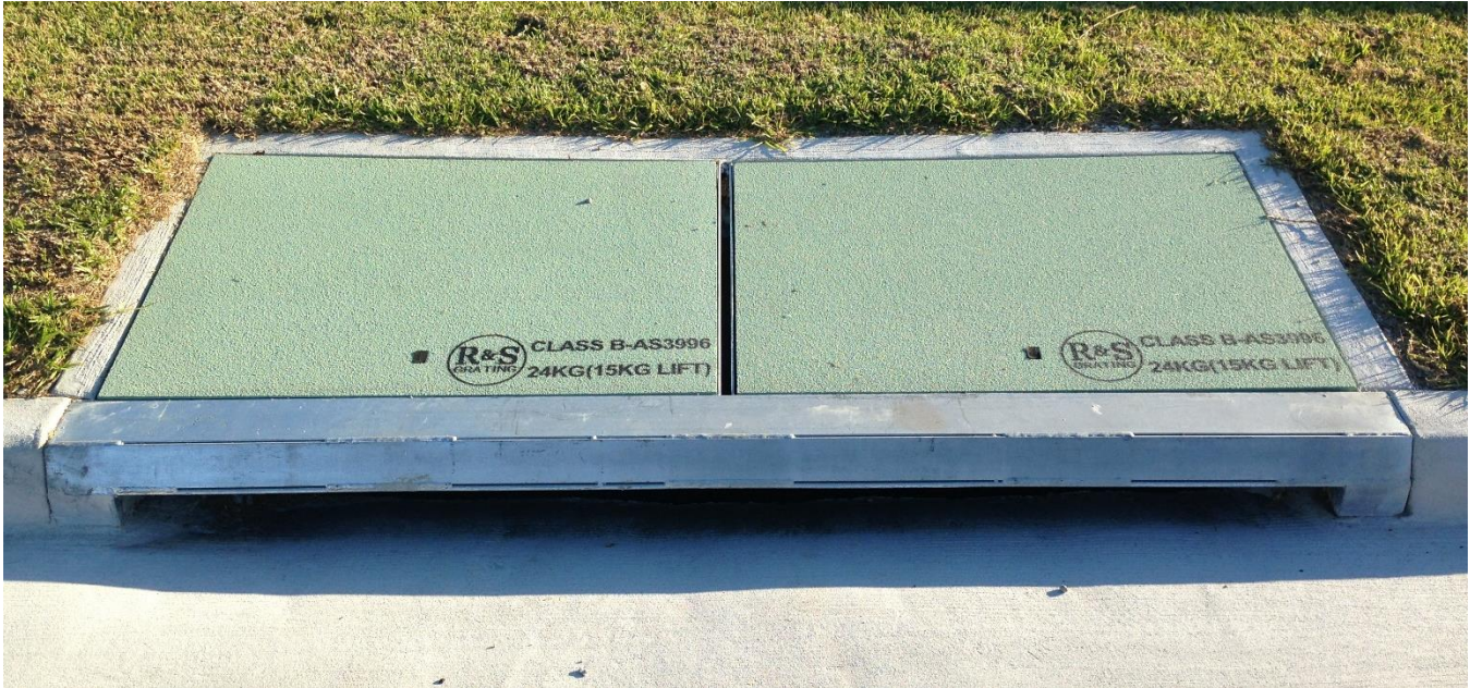
A DOUBLE SIDE ENTRY FRP INSERT WITH A FABRICATED THROATED LINTEL.
